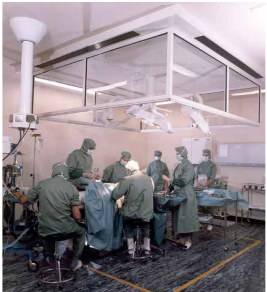
Figure 1.3 Unidirectional airflow system used on an operating theatre
