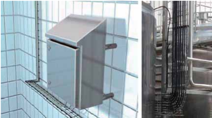
Figure 2: Cleanable arrangements of control cabinet and cabling
