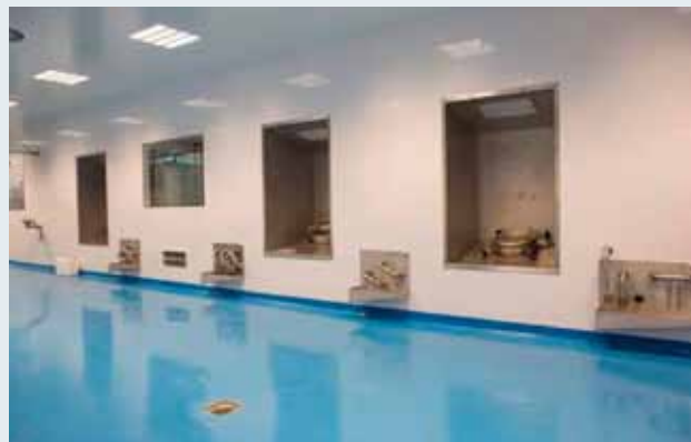
Figure 7: The clean corridor as a distribution duct towards process rooms
