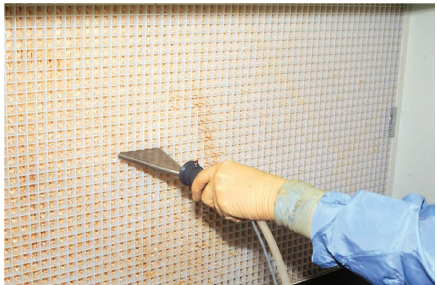
Figure D1: A probe scanning over a filter face to locate a leak
