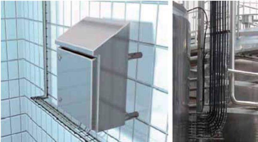
Figure 2: Cleanable arrangements of control cabinet and cabling
