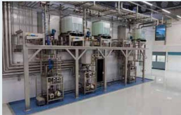
Figure 5: Process vessels and stacked raw material containers at 1st floor level in not classified basic hygiene zone as back side of Figure 5.
